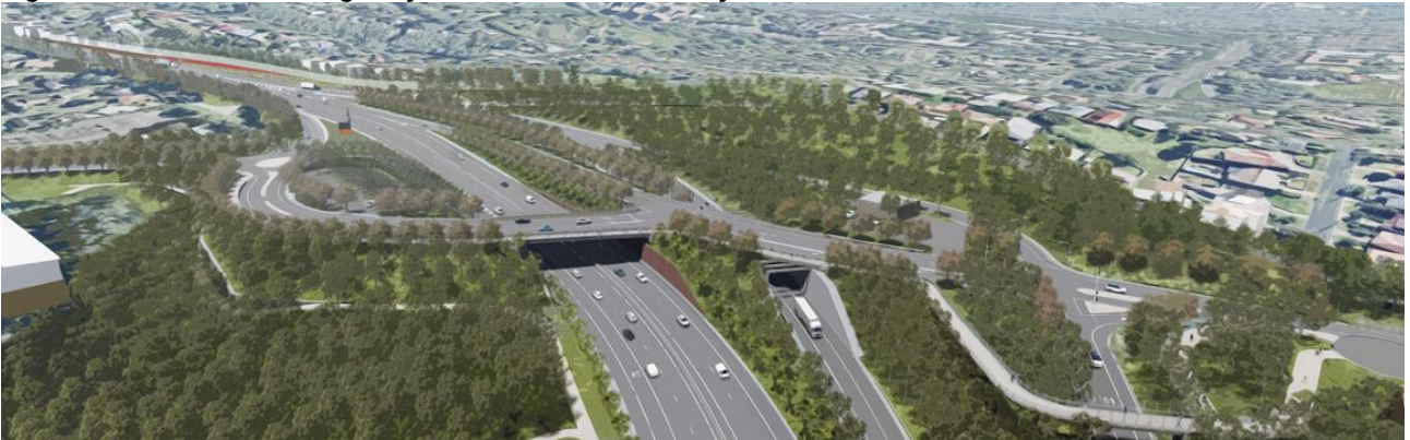
Figure 2-8: Princes Highway at Base to Mount Ousley
